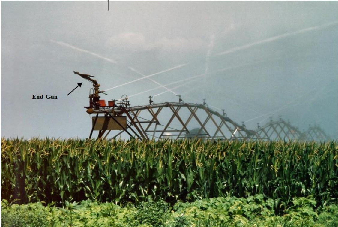
Figure 1 – A high pressure center pivot irrigation system with sprinklers on top.
